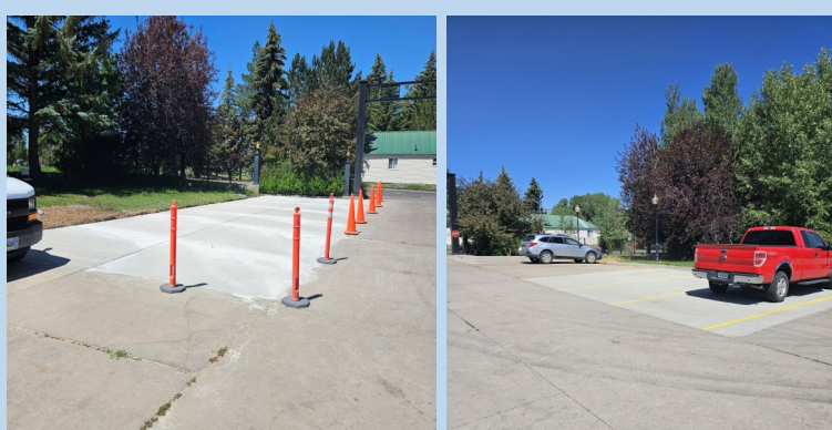
Evanston Office Parking Lot
