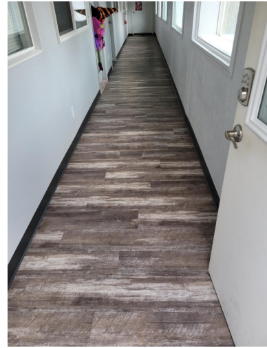
Morse Lee, Evanston, New Flooring In Back Hallway
