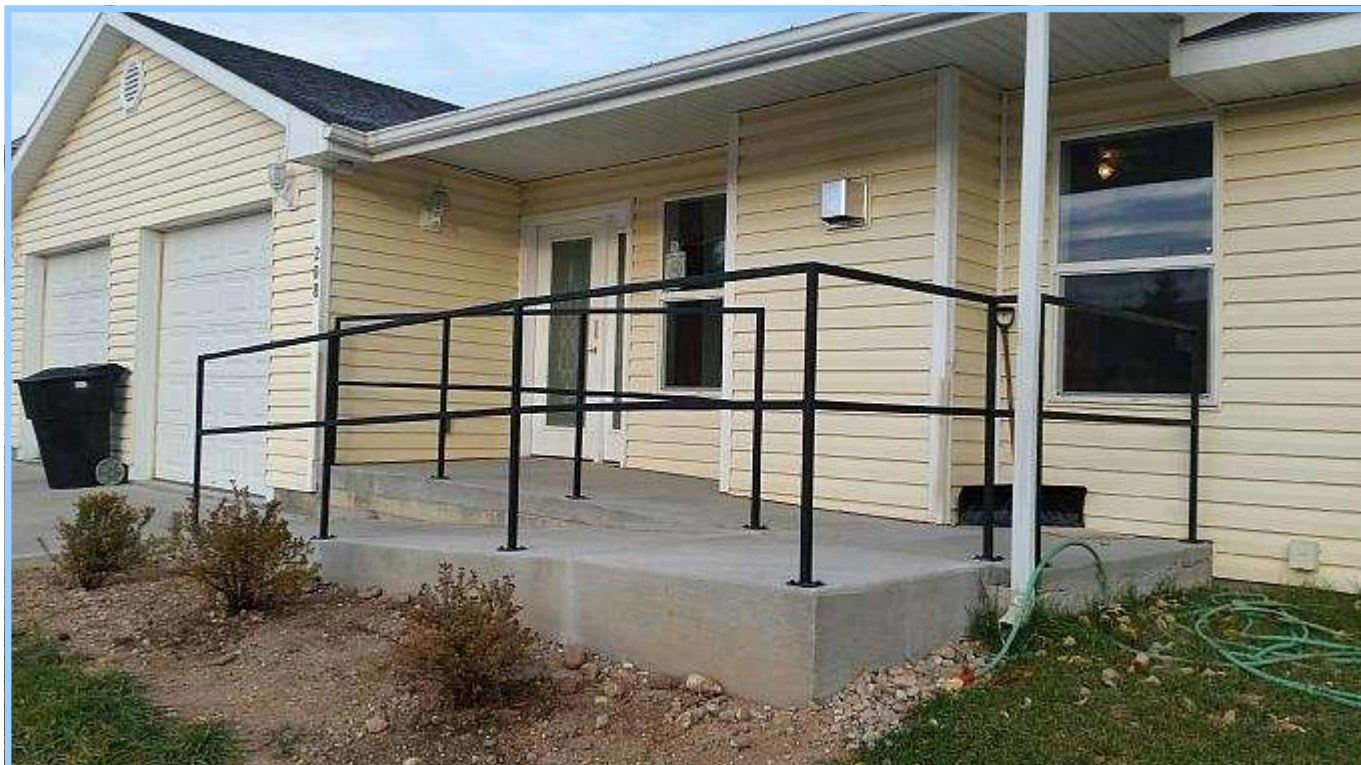
LSR'S CHAMPS RESIDENTIAL HOME GOT A NICE UPGRADE FROM A WOODEN RAMP TO A CONCRETE RAMP WITH STEEL RAILINGS.
